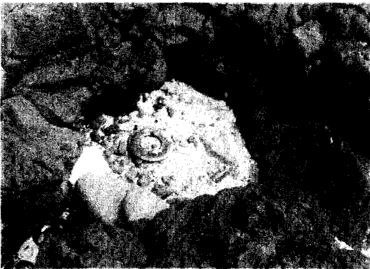
Fig 11-1. Pothole
