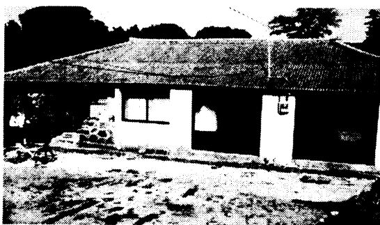
Fig. 53 A outside view of house reconstructed
